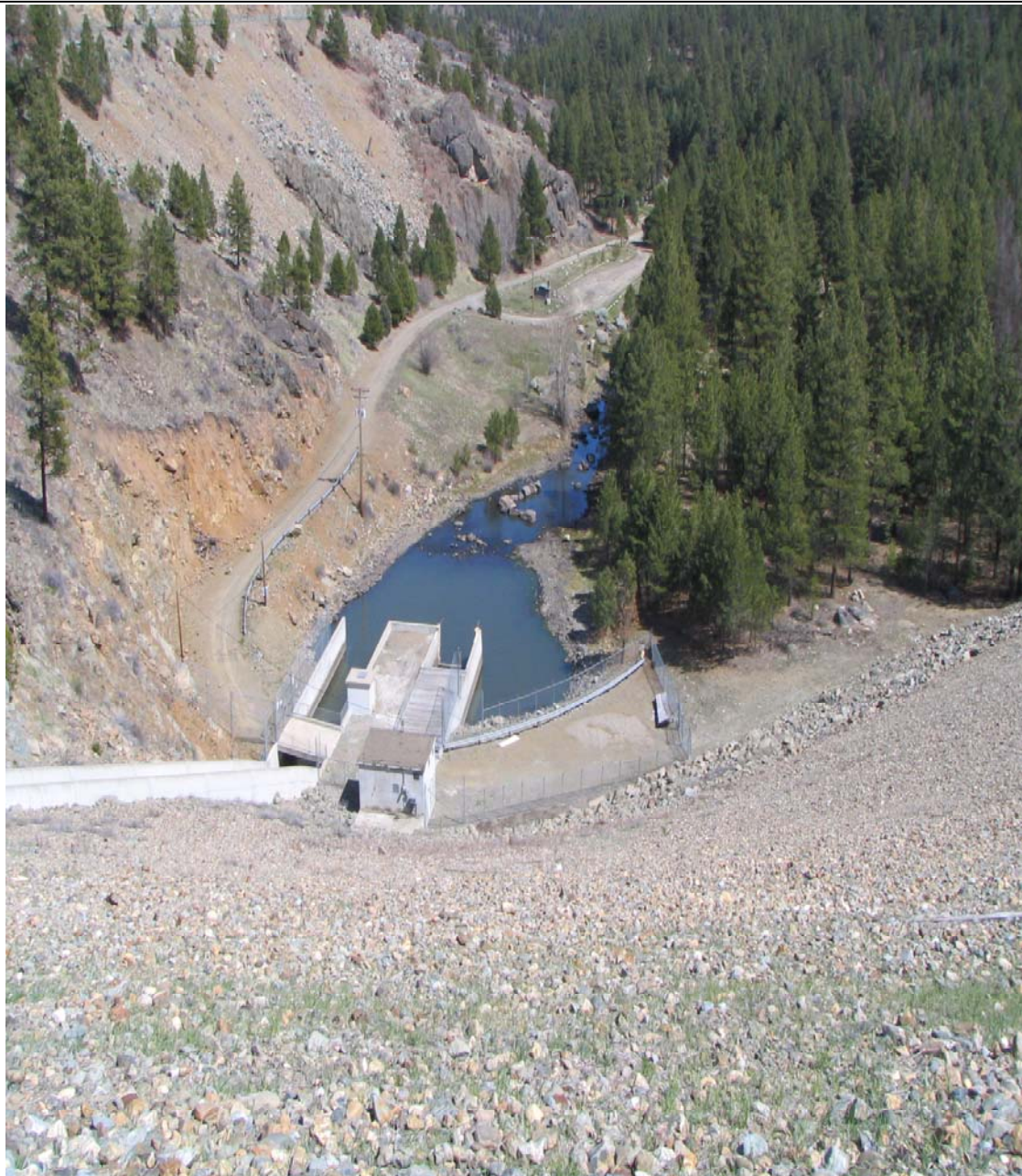
Photo 5: Control House, Spillway and Site of Proposed Power House
