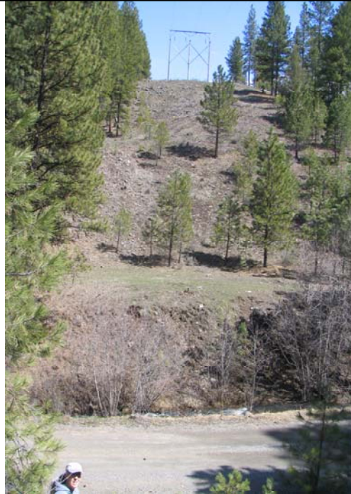
Photo 3: Idaho Power 138kv line, Black Mountain Road, Site of Proposed Substation
