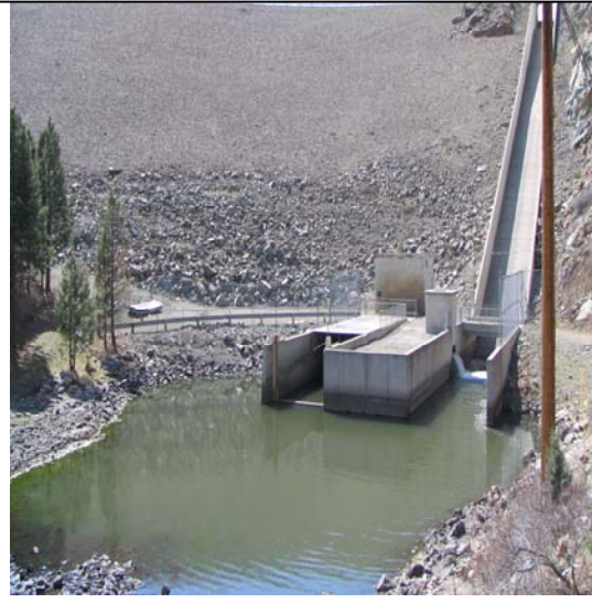
Photo 2: Mason Dam Existing Spillway, Control House and Spillway
