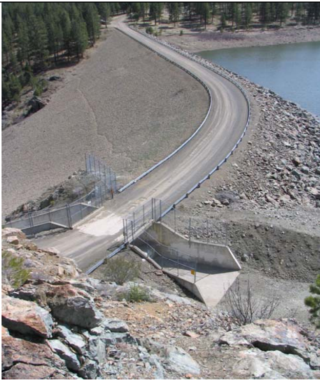
Photo 1: Mason Dam, Black Mountain Road
