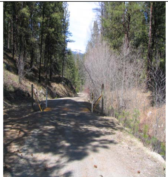
Photo 4: Black Mountain Road looking north under IPC 138 kv line
