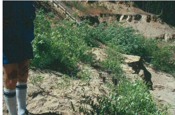
**This brush box stabilized the toe of this slide even before the willow became established, and then vegetated the slide.**
