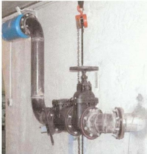
*The air intake system and valves for the draft tube aeration system at the 18-MW Lloyd Shoals plant take air from the upstream bearing gallery and feed it to the draft tubes to increase dissolved oxygen in the water.*
