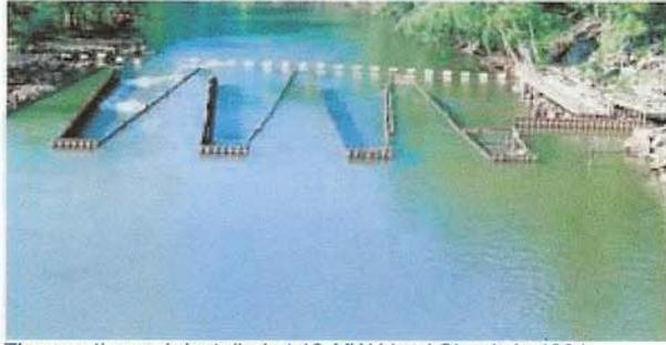
*The aerating weir installed at 18-MW Lloyd Shoals in 1991 increased downstream dissolved oxygen (DO). However, a 1994 flood damaged the weir and significantly reduced its effectiveness. Because the new draft tube aeration system installed at the plant raises DO levels to sufficient levels, Georgia Power removed the weir.*
